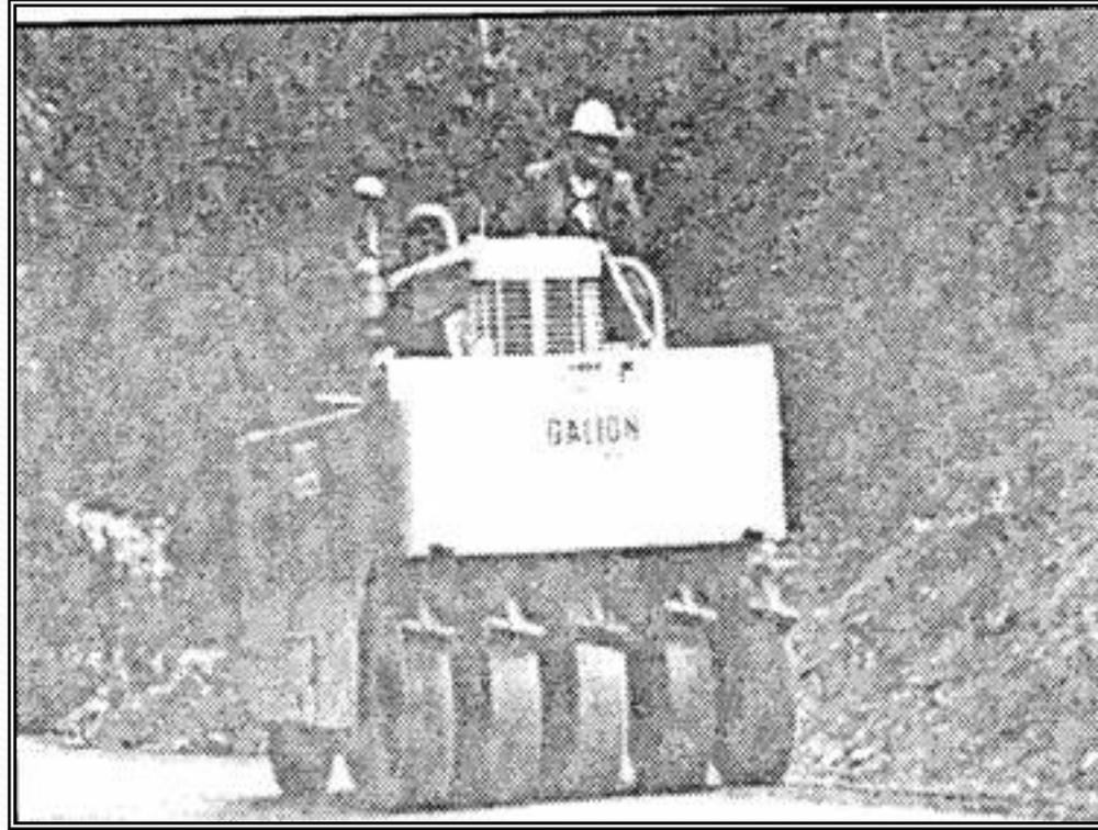
**Pneumatic roller being used to compact sand base for a highway, (courtesy of Galion Division of Dresser Industries, Inc)**
